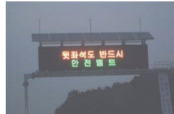
Door-Style Road Light Sign and Solar System Application
